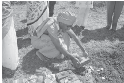
Flagging off construction at the mission site, Bangalore
